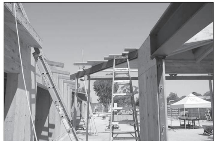
Looking north in the breezeway between the new Town Hall (on the right) and City Hall (on the left). The roof overhang is supported by ipe wood rafters (darker color) which should last forever in this coastal environment. □
