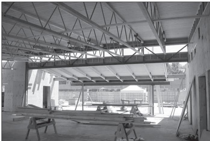
Workers laying out the roof sheathing supports for the central cupola of the new Town Hall. The picture was taken from the ground level of the Town Hall.
