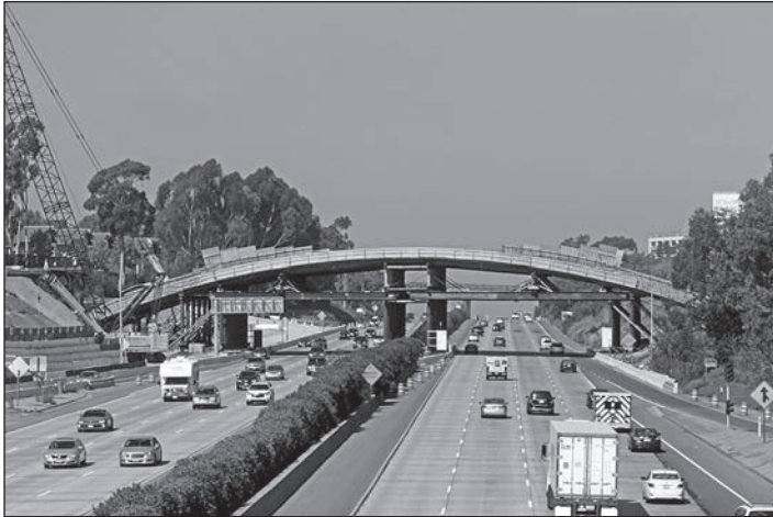
Gilman Drive Bridge. Photo Art Olson
